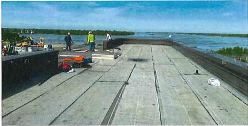
SUBR J S Clark Building Roof Replacement
