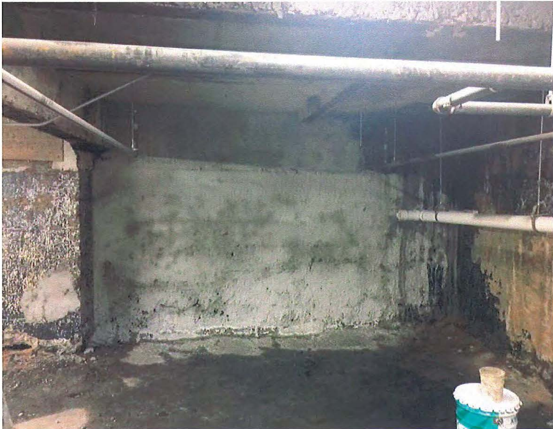
Basement waterproofing in progress
